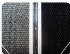
Cooling Tower Fill Before/After Cleaning
