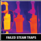
FAILED STEAM TRAPS
