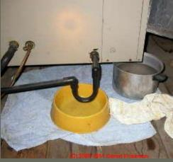
Secondary Pan: function poorly communicated sometimes drains into occupied area can cause hidden mold
