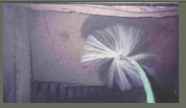
• Flex Duct: residential can tear when cleaned; cannot clean
