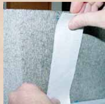
Line up tape with seam
