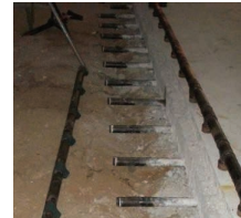
Buckley AFB protection of in slab heating
