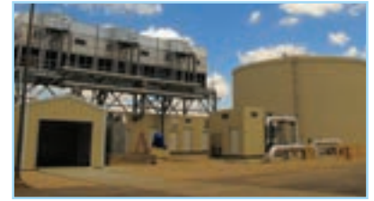
Power Plants Cleburne, TX ▶ 1.74 MG TES Tank
