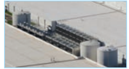
Data Centers Ashburn, VA ▶ (3) 0.50 MG TES Tanks
