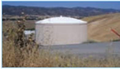
Industrial & Commercial Brooks, CA ▶ 1.37 MG TES Tank
