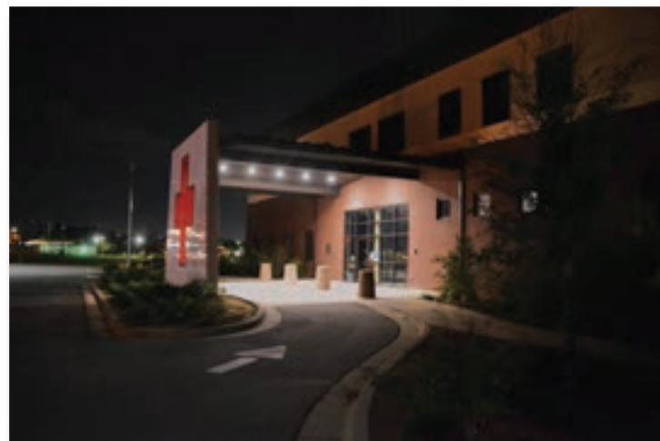
After: Retrofitting with 40W HyLite LED Lotus Lamps
