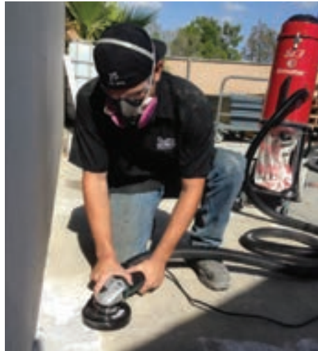
Shroud used with an S-13 curbs dust.
