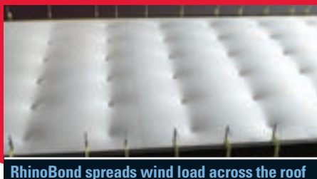
RhinoBond spreads wind load across the roof
