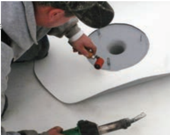
Hercules style retrodrains are available with PVC and TPO coated flange for direct membrane attachment.
