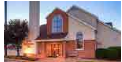
Residence Inn Harrisburg, PA
