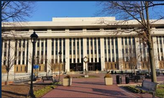
Prince George's County Administration Building; Marlboro, MD
