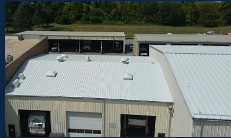
FrederickCounty Warehouses Frederick, MD
