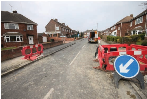
Lead Service Lines - No Road Closure
