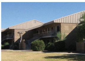
Davis AFB pinhole leaks copper
