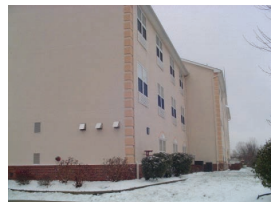
Fort Knox potable water corrosion prevention
