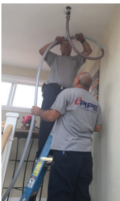
Fire Sprinkler Suppression Systems
