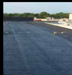
ASPHALT/BUR/ GRANULAR CAP SHEET
