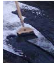
Reinforcement fabric embedded into UNIFLEX non-fibered asphalt emulsion
