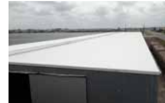
Gravel BUR restored with UNIFLEX asphalt emulsion system and top coated with premium white reflective finish coat
