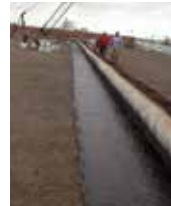
Reinforcement fabric embedded into UNIFLEX non-fibered asphalt emulsion
