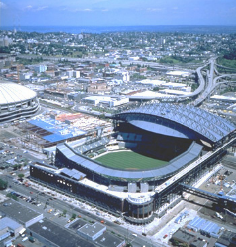
Sensors and structural integrity monitoring of CenturyLink Field Roof Truss
