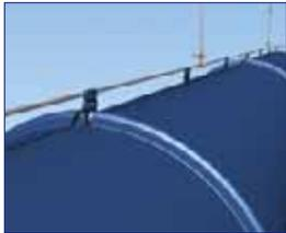
All-in-One on an H-rail. Ducts on H-rails are quickly installed or taken down for washing.
