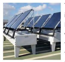
ThermX integrates into new and existing HVAC/R systems and works by harnessing free thermal energy from the sun to massively reduce
