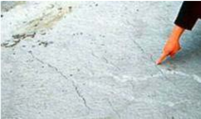
Plastic Shrinkage Cracks
