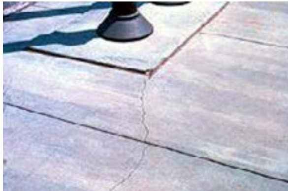
Drying Shrinkage Cracks
