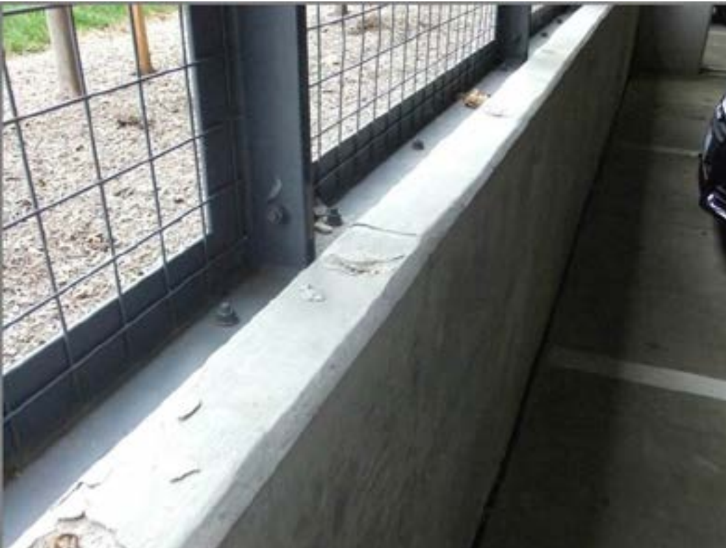
Concrete Spalls (rebar cover issue)
