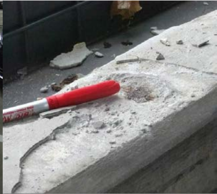
Concrete Spalls (rebar cover issue)
